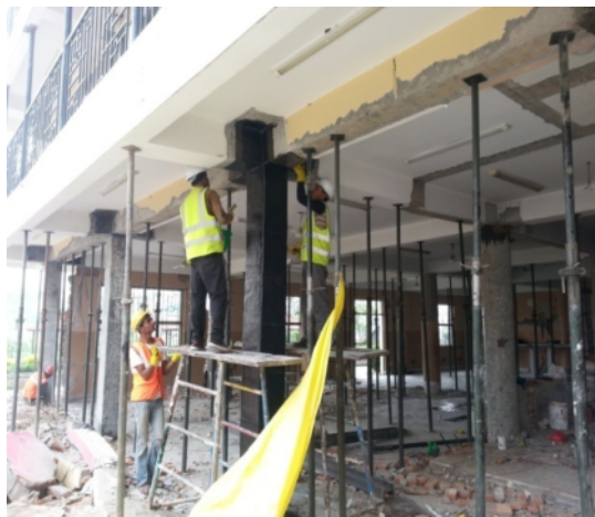
Fig 14: Carbon Fiber Jacketing
