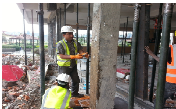
Fig 22: Epoxy Mortar with Epoxy Injection
